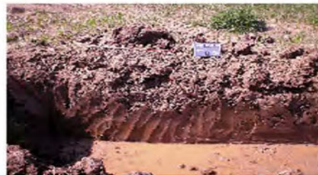
Plate 3 – Trench 1 section, looking southwest
